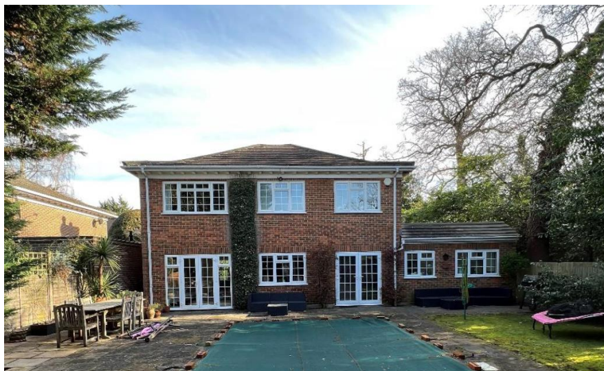
Figure 3: Rear of the property
